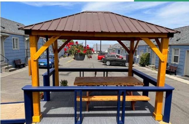
Thank you Nor'Wester Rotary Club of Port Angeles for installing a stunning new gazebo at the Dawn View Court.
