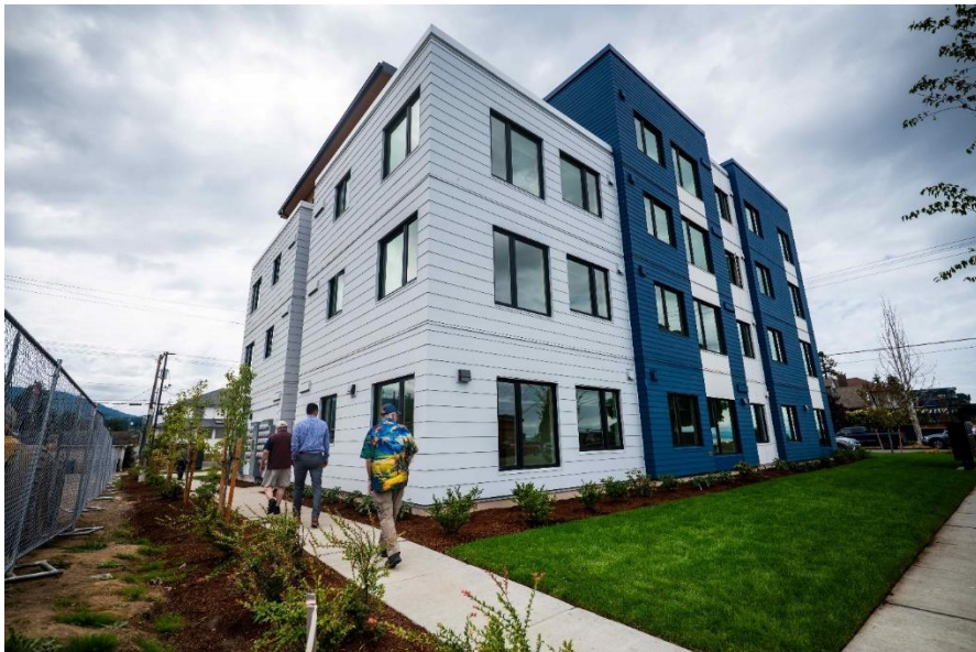
Exterior View of North View Permanent Supporting Housing in Port Angeles, WA.
